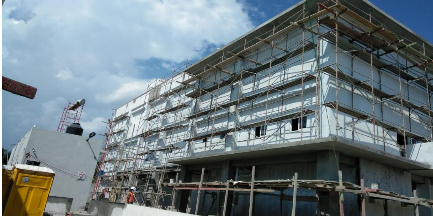
HOSPITAL MUNICIPAL DE BOCA CHICA, SANTO DOMINGO
