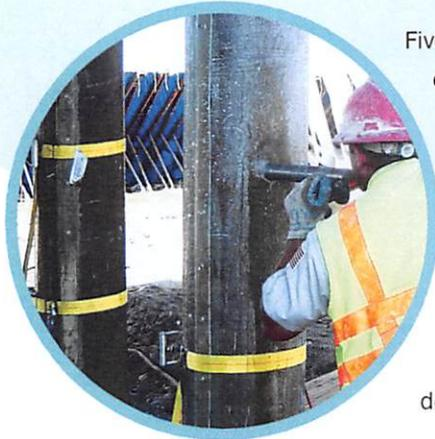
Five Star® PileForm™ F FRP (Fiberglass Reinforced Plastic) pile rehabilitation jackets meet and exceed marine engineering specifications for use in hostile marine environments where exposure to ice, floating debris, chemical pollution, oils, acids, salt water and tidal action may occur. PileForm™ F FRP Pile Rehabilitation Jackets are available in thicknesses of 1/8" nominal to 1/2" minimum, and they can be translucent, pigmented or gel coated to any specified color.
